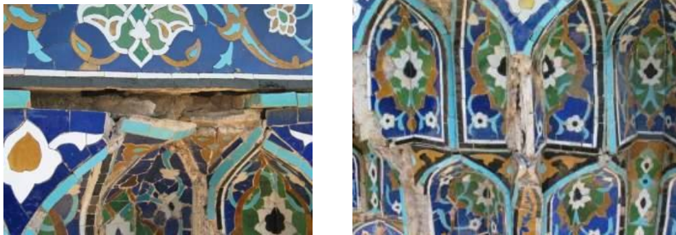
Figure 17 & 18 - Tile layer separation from gypsum bed (Writer)
