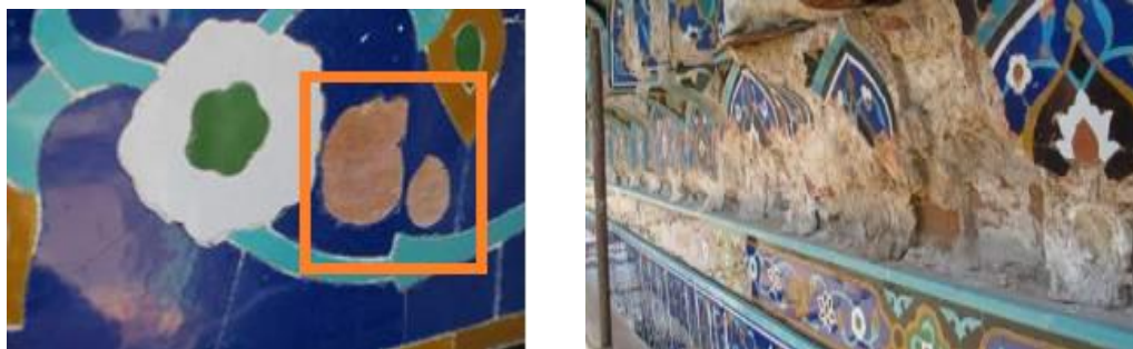
Figure 20 - Tile drop and disappearance of bed sheet (writer)
