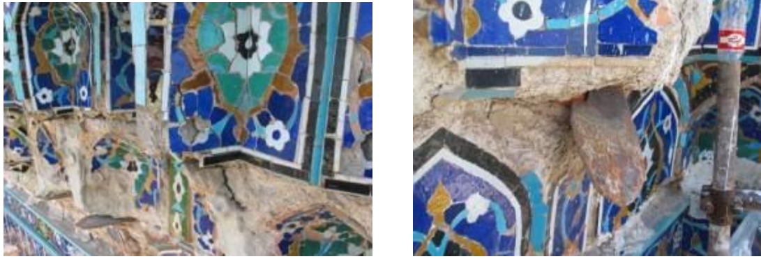
Figures 15 and 16 - Laying Metal Plates (Writer)
