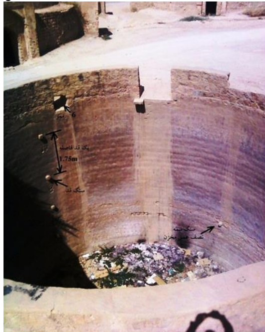
Figure 4. component and inner part of reservoirs.
